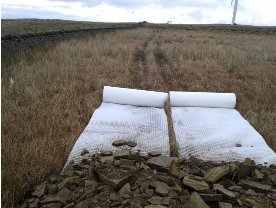
Plate 13: Semi-permeable geotextile layer
