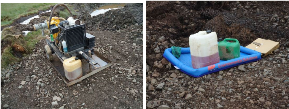
Plate 12: Examples of drip trays and bunds
