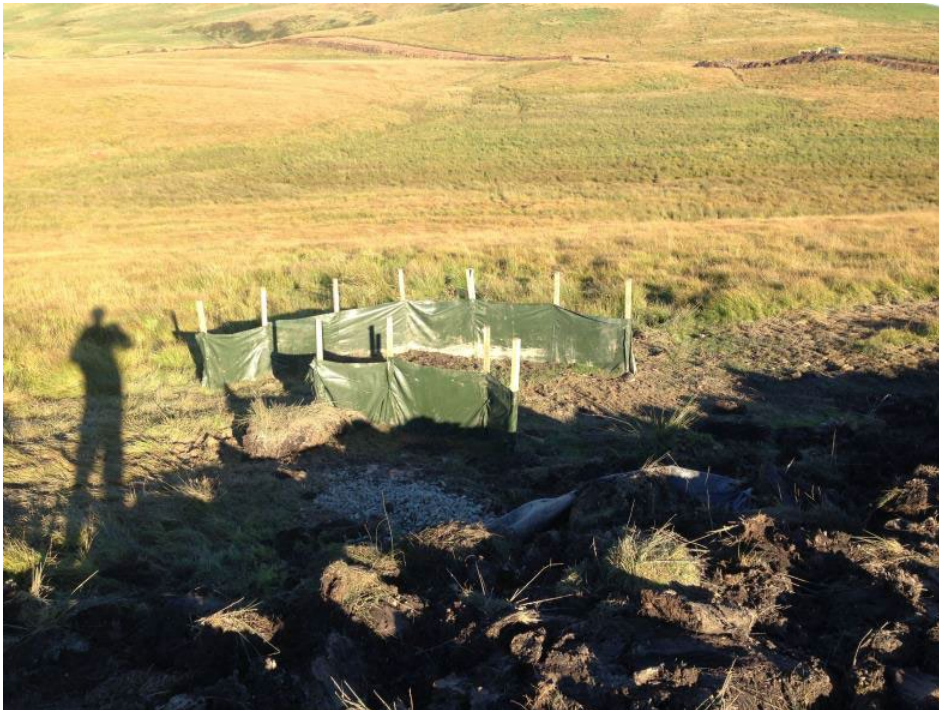
Plate 1: Typical silt fencing
