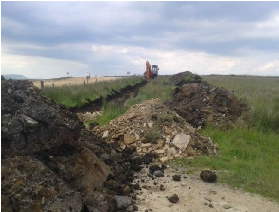
Plate 14: Typical overburden stockpile measures
