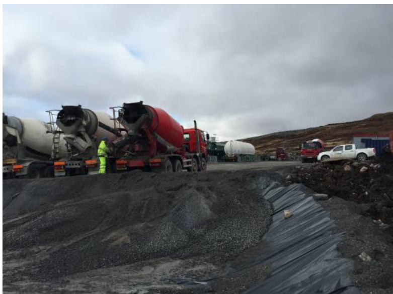
Plate 10: Typical concrete wash-out facility
