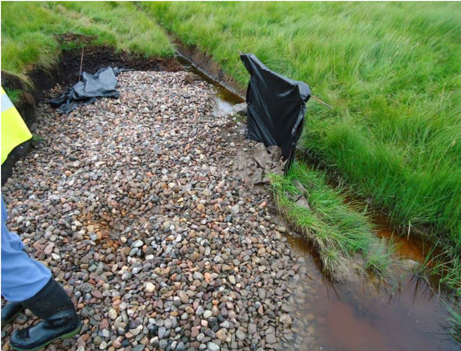
Plate 2: Typical silt traps
