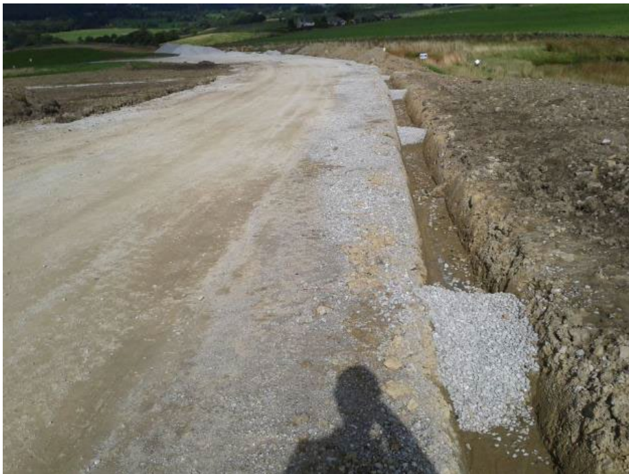
Plate 4: Typical check dams – to be installed in drainage ditches adjacent to roads
